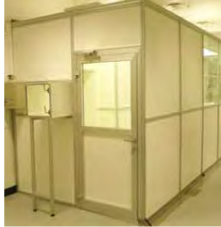
SBM entrance with material pass trough
