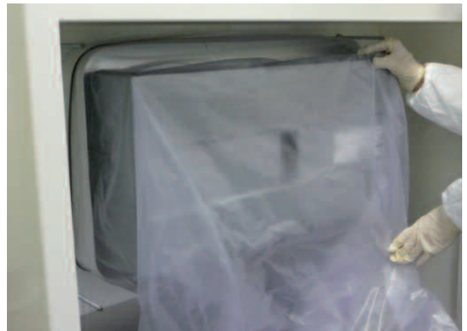
Filter with Bag-in Bag-out system
