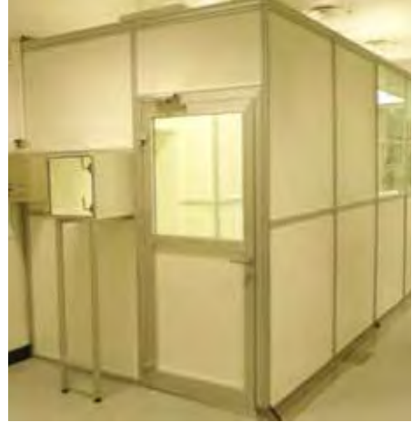
SBM entrance with material pass trough
