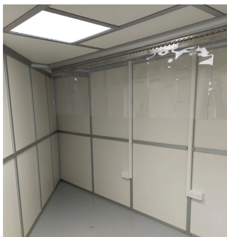
HPL walls with example of a 40° angle
