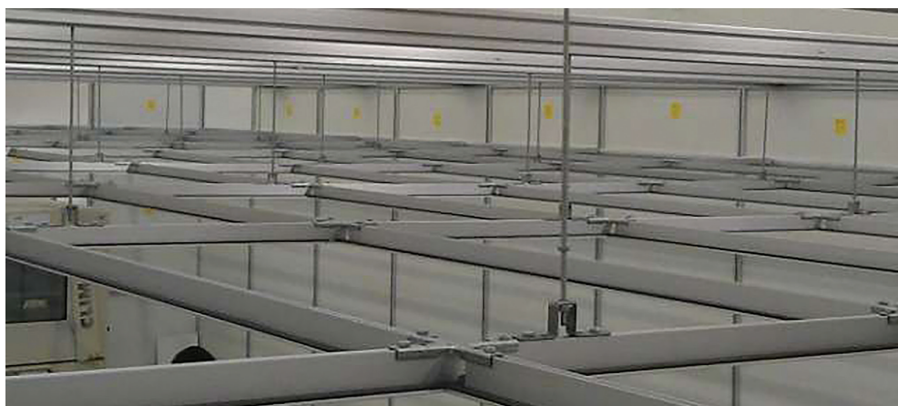
View of the ceiling of an SBM, self-supporting construction. T-Bar ceiling suspended from the SBM structure
